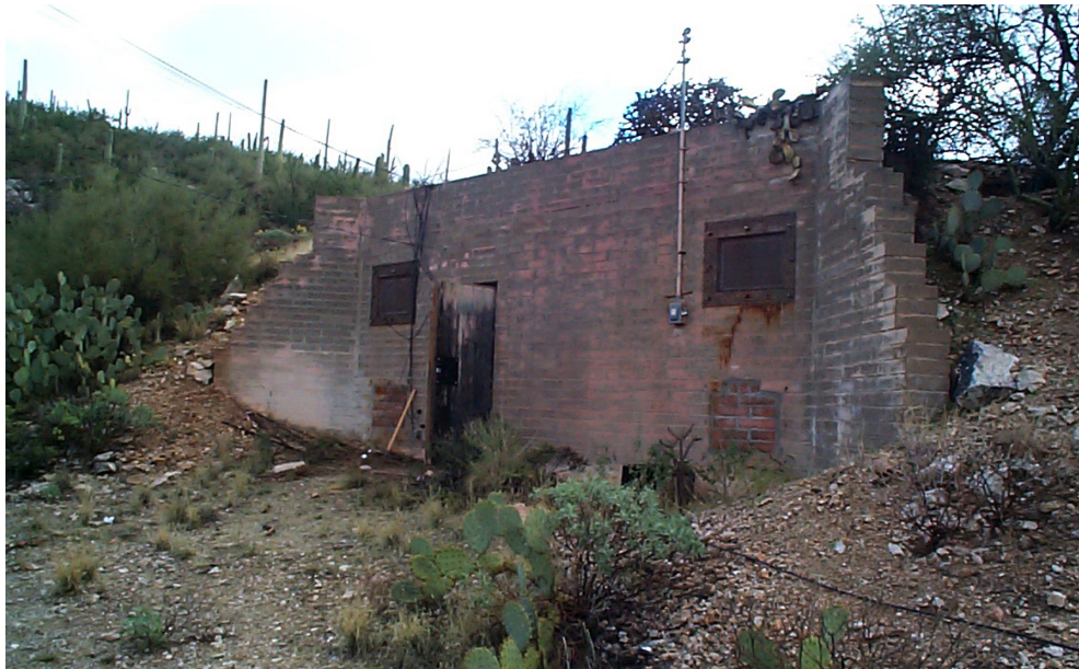
Figure 5: The seismic vault for TUC where the digitizer (Ref-Tek 72A-06), disk and battery are located. Commercial power is used to charge the 12-volt battery operating the data logger.
